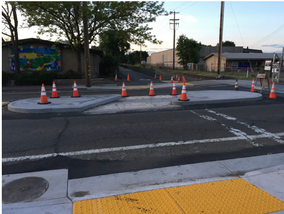
IN-PROGRESS INSTALLATION OF NEW PEDESTRIAN SAFETY ISLAND AT GOBBI STREET RAIL TRAIL CROSSING
