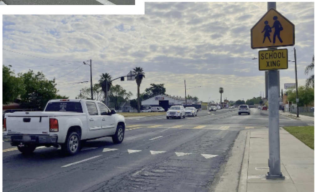
ABOVE: A high-visibility yellow crosswalk with an overhead flashing pedestrian signal on West Inyo Avenue (SR-137) alerts drivers of students crossing in the area.
