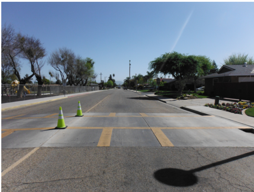
Raised crosswalk, a typical engineering improvement suggestion for school area
