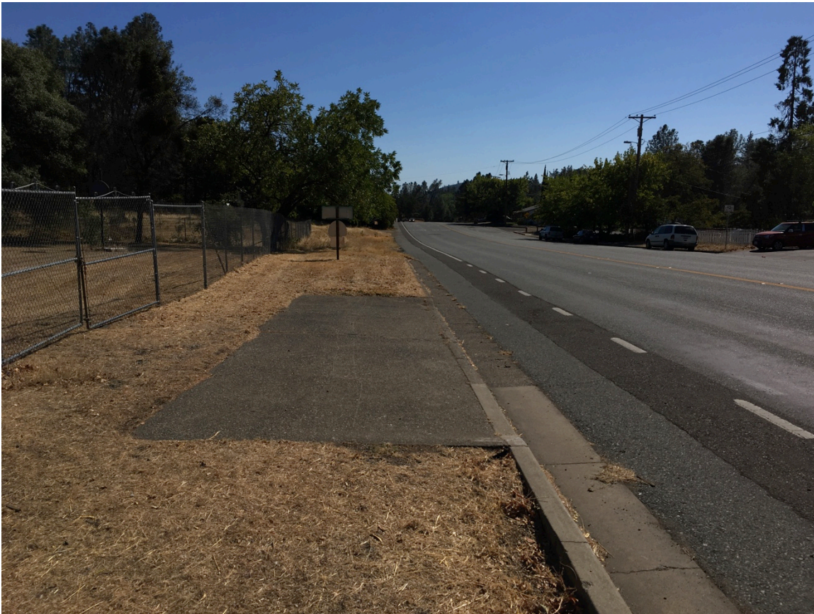
STRETCH OF LAKE BOULEVARD (50 MPH POSTED SPEED LIMIT) LACKING SIDEWALKS THAT STUDENTS REGULARLY TRAVERSE ON FOOT TO/FROM SCHOOL, HOME, AND NEIGHBORHOOD CONVENIENCE STORE.
