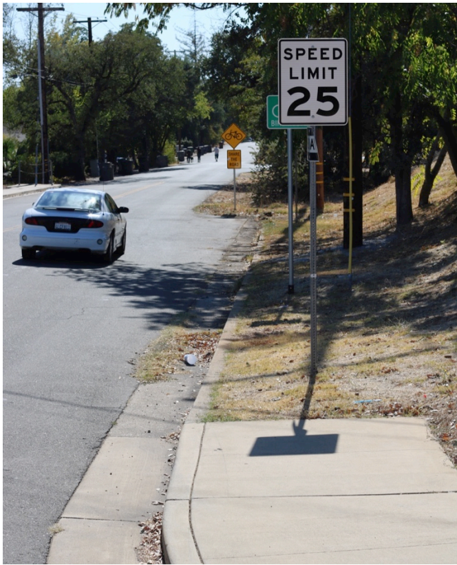
SIDEWALK ABRUPTLY ENDS DURING WALKABILITY ASSESSMENT.
