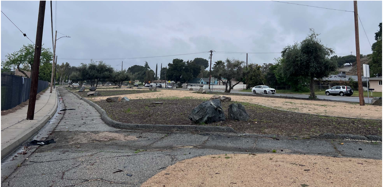
ABOVE: Just south of the Arrowhead Elementary School campus, debris and litter pose a risk for those walking or biking to school.
