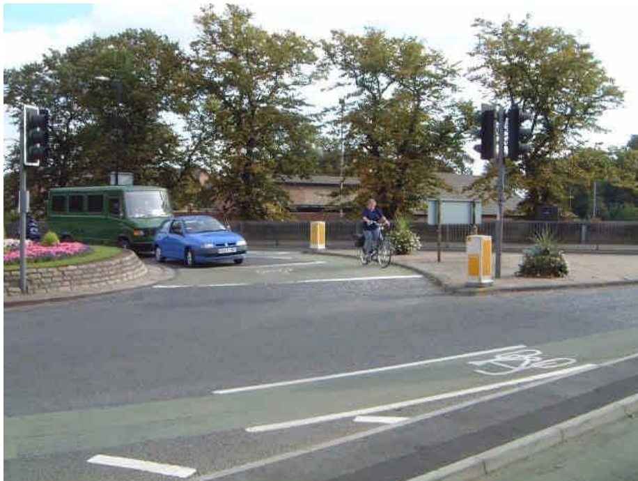
Figure 29: Signalized Roundabout York, England
