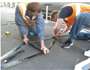
Technicians installing temporary inductive loop detectors.
