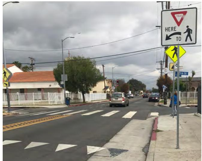
*Left: Speed humps and low speed posted speed limit on northbound Grape Street. Right: High-visibility pedestrian crosswalk at the intersection of Wilmington Avenue and 105th Street.*
