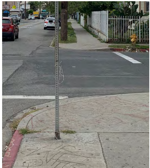
Left: Lack of curb ramps on alleyway. Right: Lack of truncated dome and accessibility features for visually impaired pedestrians at East 25th Street and Hooper Avenue.
