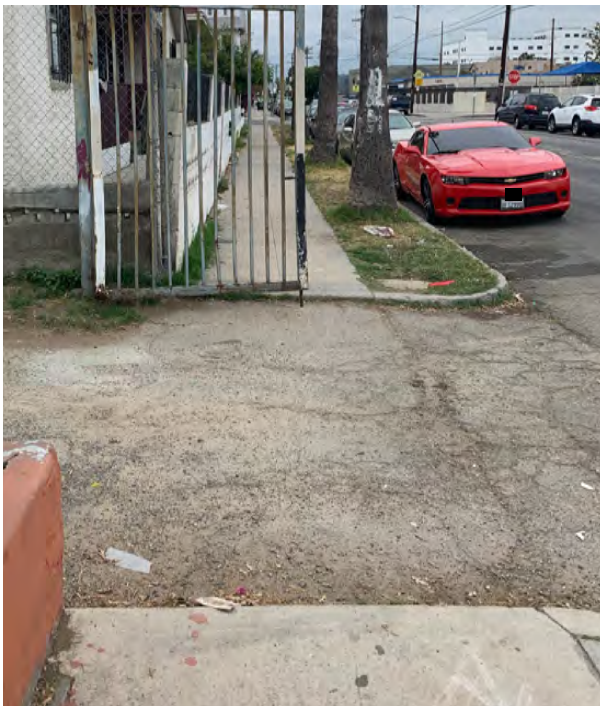
Left: Lack of curb ramps on alleyway. Right: Lack of truncated dome and accessibility features for visually impaired pedestrians at East 25th Street and Hooper Avenue.
