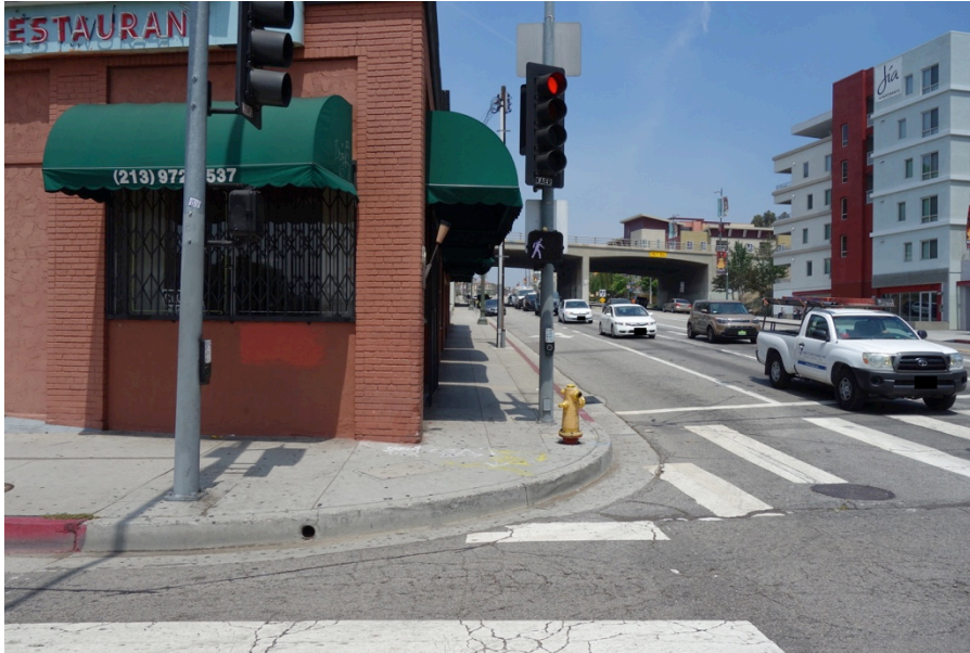
HIGH CURB AND LACK OF CURB RAMP AT N. BROADWAY AND CESAR CHAVEZ AVENUE
