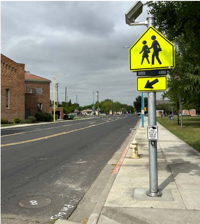
ABOVE: A rectangular rapid flashing beacon at Draper Street and Sierra Street (SR-201) signals drivers that pedestrians are crossing.
