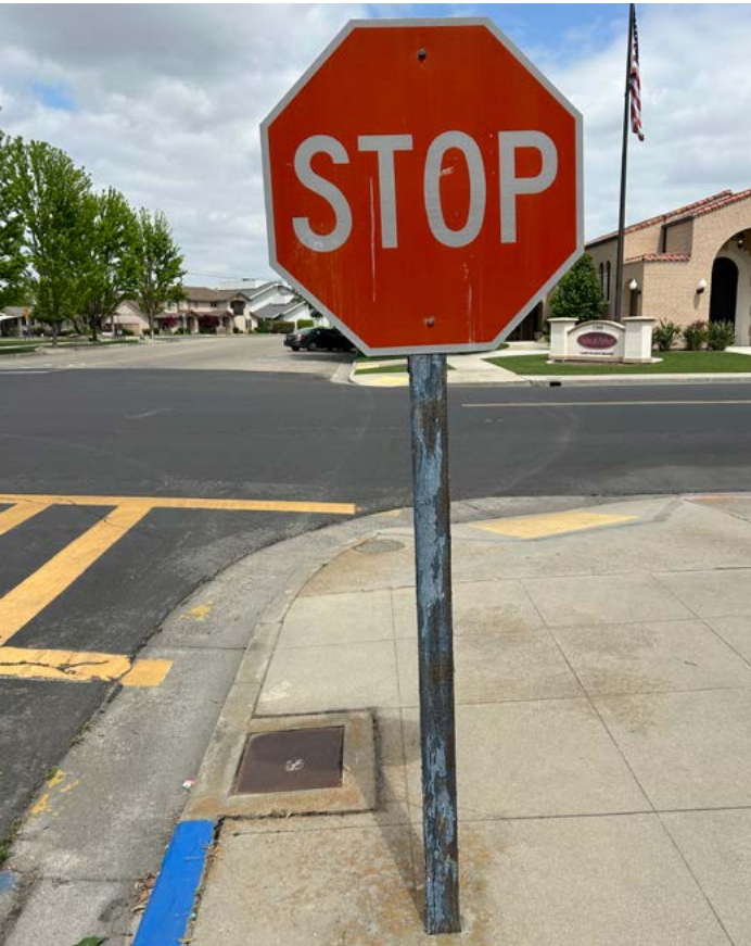
ABOVE: Shorter than standard height stop signs at the Ellis Street / Lincoln Street intersection and at the Ellis Street / Sierra Street (SR-201) intersections, which need to be more visible.
