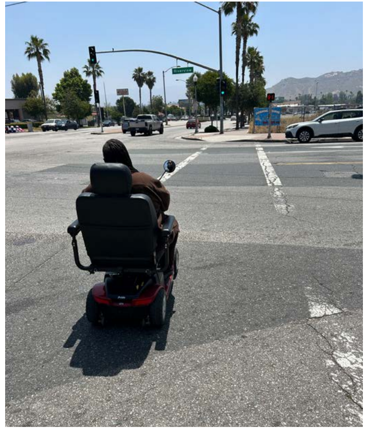
ABOVE: Faded crosswalk paint at Mission Boulevard/ Riverview Drive intersection crossing.
