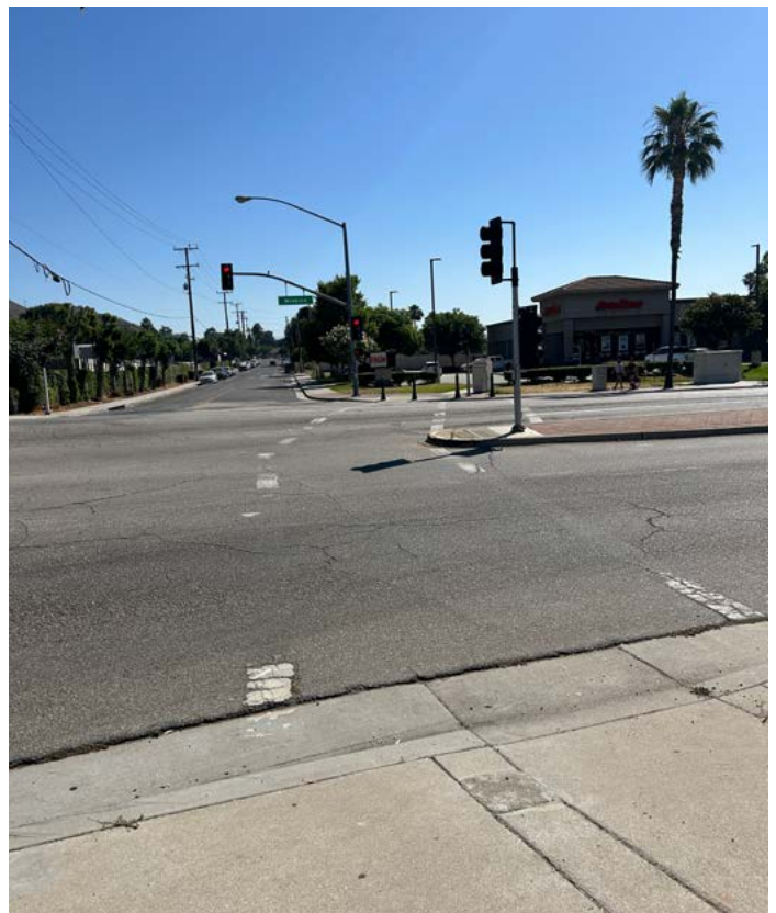
ABOVE: The east-west painted crosswalk at the intersection of Mission Boulevard/Riverview Drive is faded and deteriorated.
