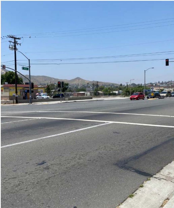
ABOVE: The painted crosswalk at Mission Boulevard and Pacific with no pedestrian refuge island.
