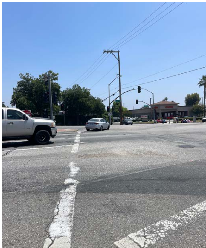
ABOVE: There is no marked east-west crosswalk on the north side of the Riverview Drive/Mission Boulevard Intersection, causing safety concerns for those crossing the street.
