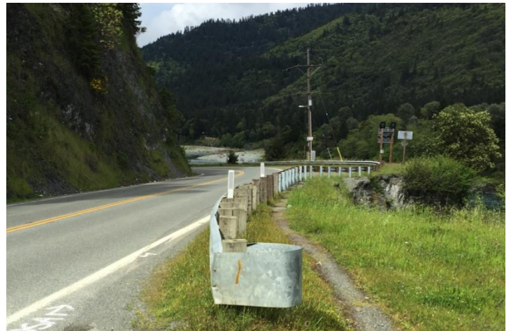
CLEARLY WORN PEDESTRIAN PATHS ALONG THE SIDE OF SR-96 IN THE BLUE SLIDE SECTION; ERODING SECTIONS OF THE INFORMAL PATH EXPOSE PEDESTRIANS TO DANGEROUS CONDITIONS
