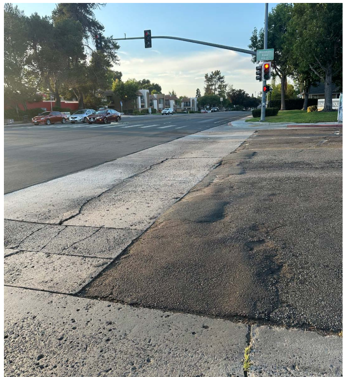
ABOVE: Faded and deteriorated crosswalk lines in the north-south direction on Camino Ruiz, at the intersection of Camino Ruiz/Westmore Road.
