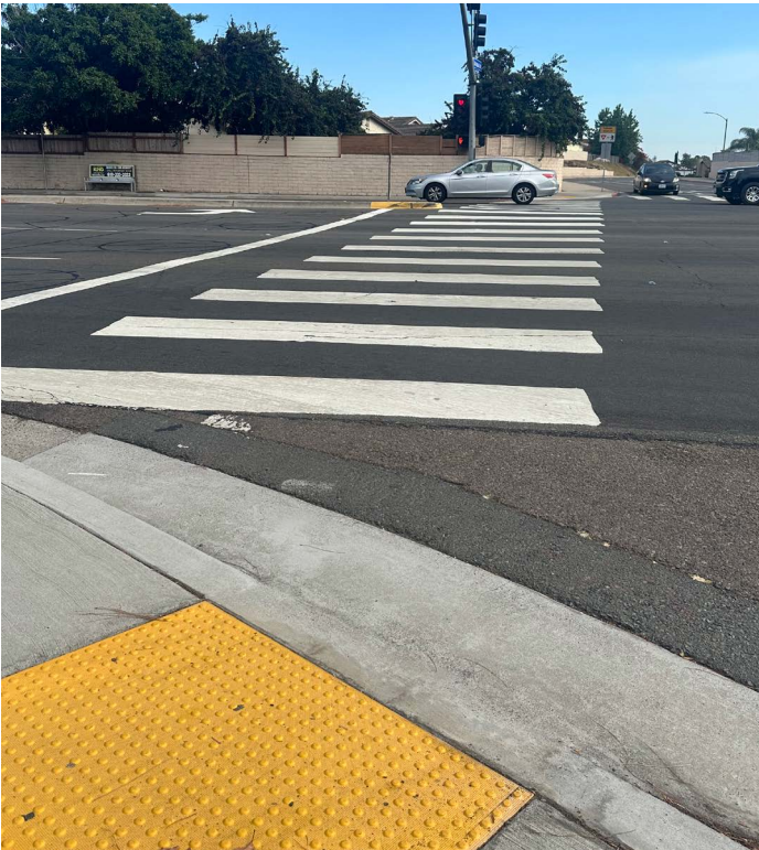
ABOVE: At the intersection of Mira Mesa Boulevard/Aderman Avenue, the sidewalks are well maintained and have truncated domes for accessibility and the north-south crosswalks are freshly painted.
