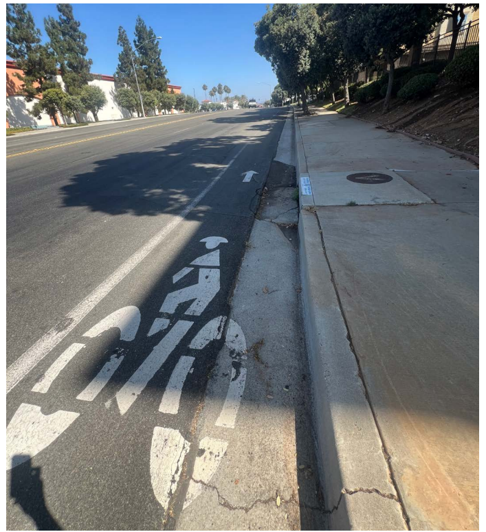
ABOVE: The cracked, uneven pavement within the Class I bike lane markings near the northeastern corner of the Hillery Drive/Westview Parkways which poses a tripping hazard to bicyclists.
