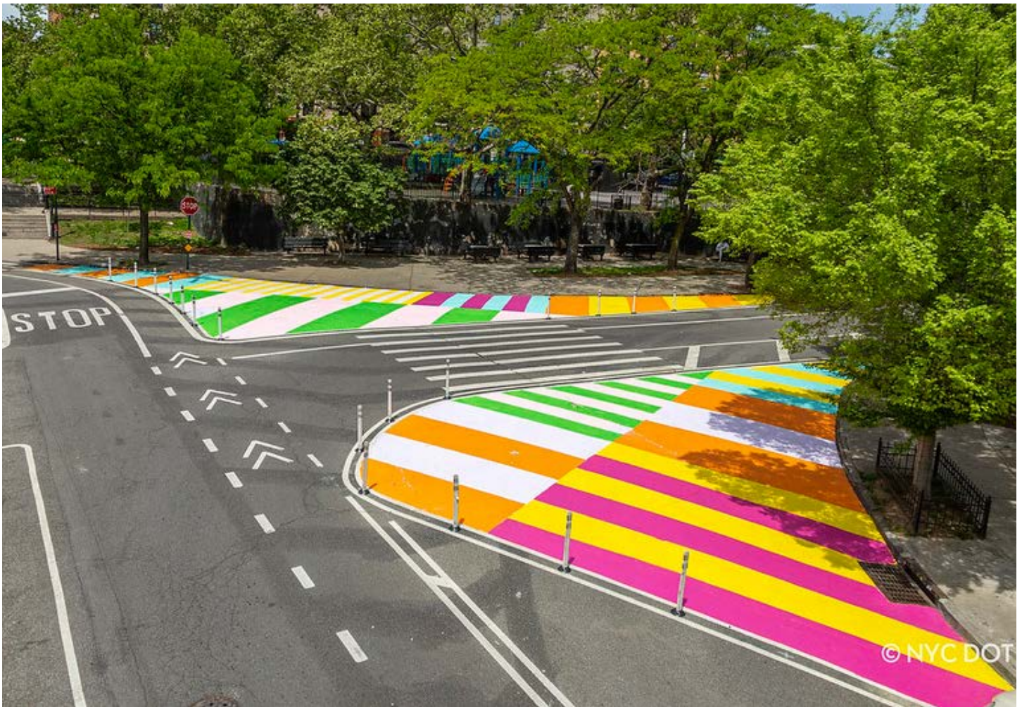
ABOVE: Image is an example of a Quick-Build, consisting of a multi-colored corner wedge with soft posts. Source: NYC Asphalt Art Activations: “Birds – Eye View” by Mary Carter Taub. Photo credit: NYC DOT. Photo credit: NYC DOT.
