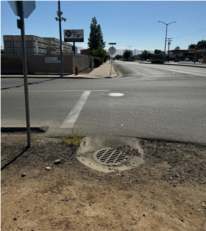
ABOVE: There is a lack of high-visibility road markings and crosswalks at the Park Boulevard/Anchor Avenue intersection.
