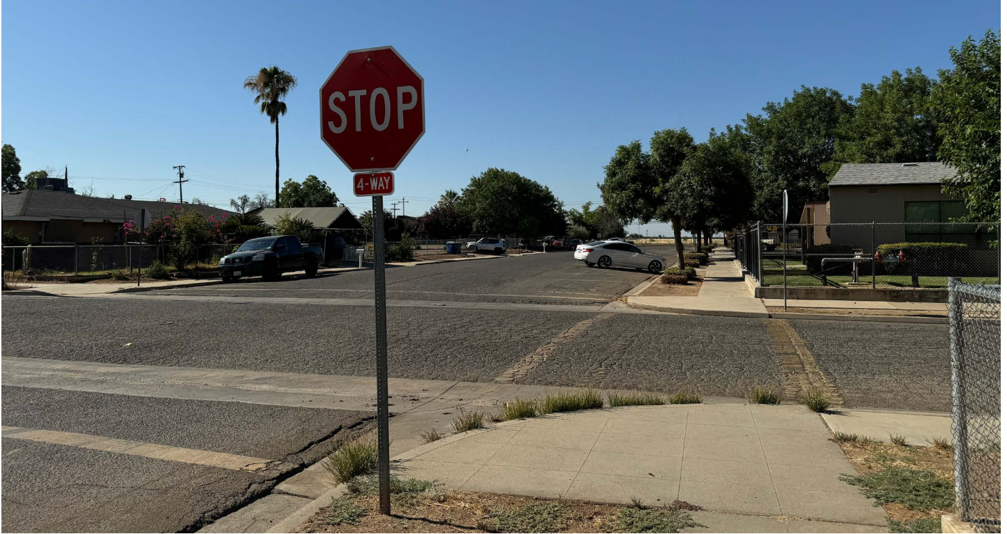
ABOVE: The four-way stop adjacent to Sheridan Elementary School at the 9th Street/J Street intersection demonstrates faded crosswalk markings, severe cracks, and potholes.
