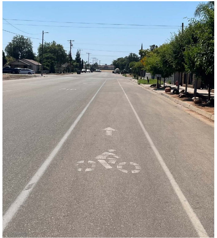
ABOVE: Designated bike lanes like the Class II bike lanes located on G Street support biking and rolling.
