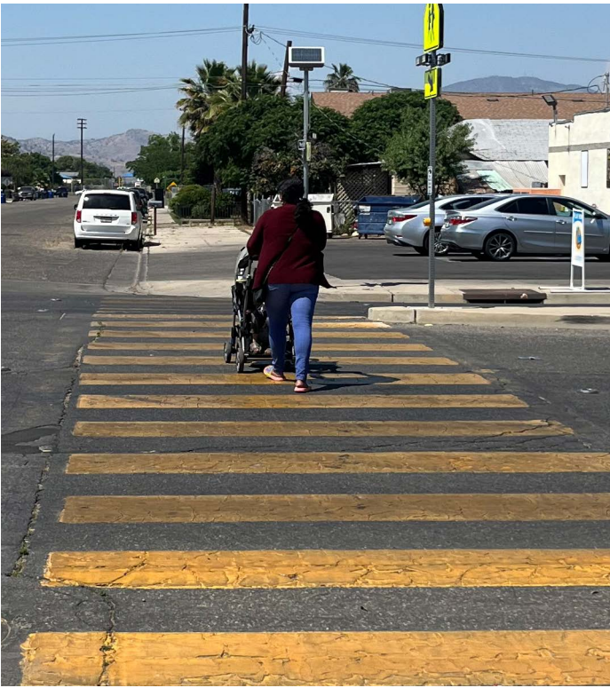
ABOVE: A pedestrian walks with a child in a stroller northbound on Park Boulevard across a high visibility yellow continental crosswalk supported by RRFBs.
