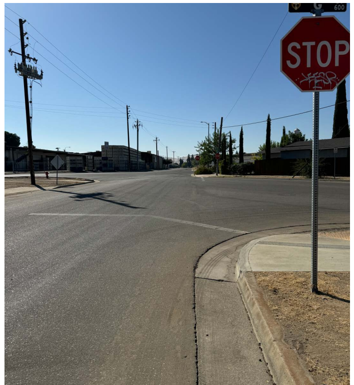
ABOVE: The three stop signs in close proximity to each other at the G Street/West Railroad Avenue/South Jacobs Center Street intersection, near the Orange Cove Branch Library, create confusion.
