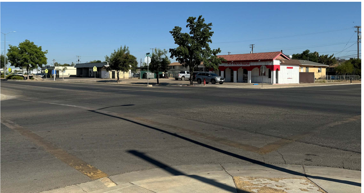
ABOVE: South Jacobs Center Street and Park Boulevard intersect at a four-way stop in the center of Orange Cove. This central intersection lacks visible road markings and high-visibility crosswalks. The yellow standard crosswalk marking paint is faded.
