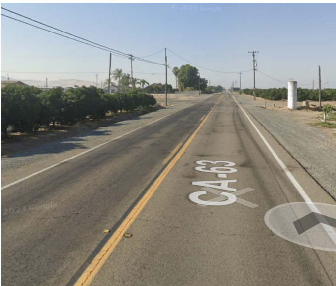
ABOVE: Pedestrian Crash Location: On South Hills Valley Road (State Route 63).
