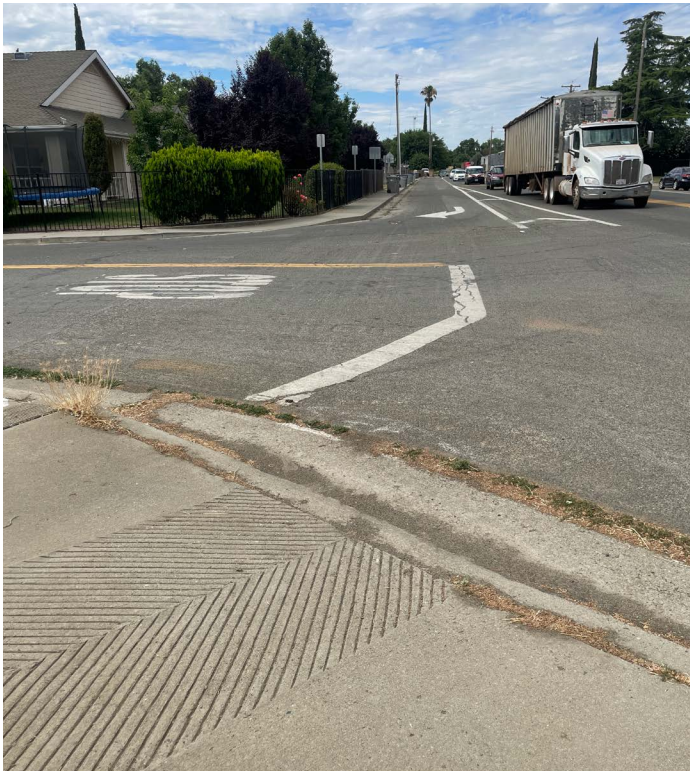
ABOVE: The Road 116/Locust Street (SR-113) intersection was identified as a key area of concern for people walking, biking, or rolling.
