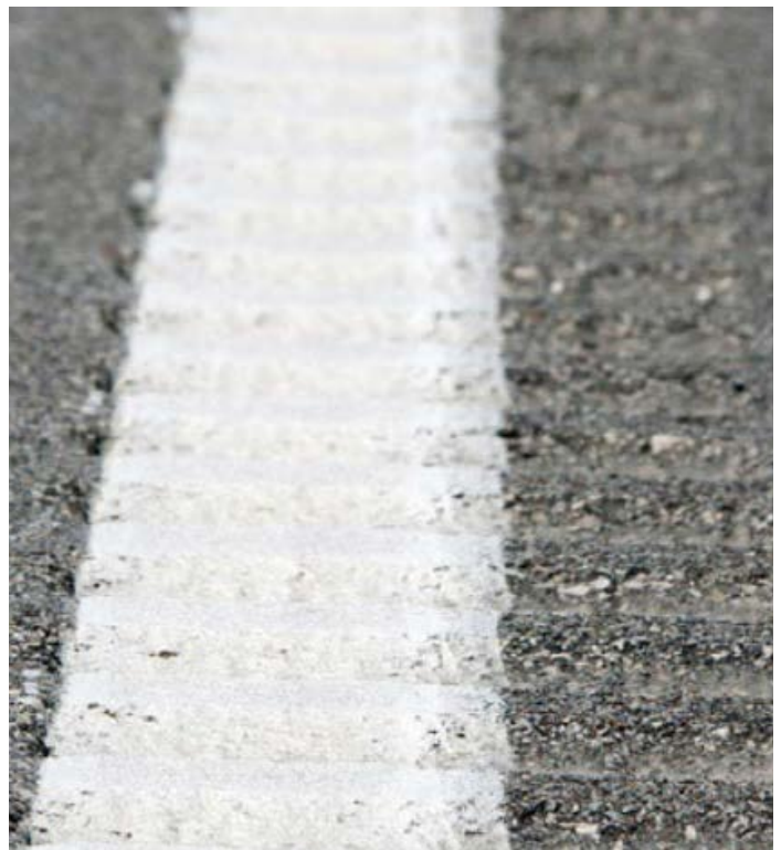
ABOVE: Example of an edge line rumble strip. Source: Missouri DOT.
