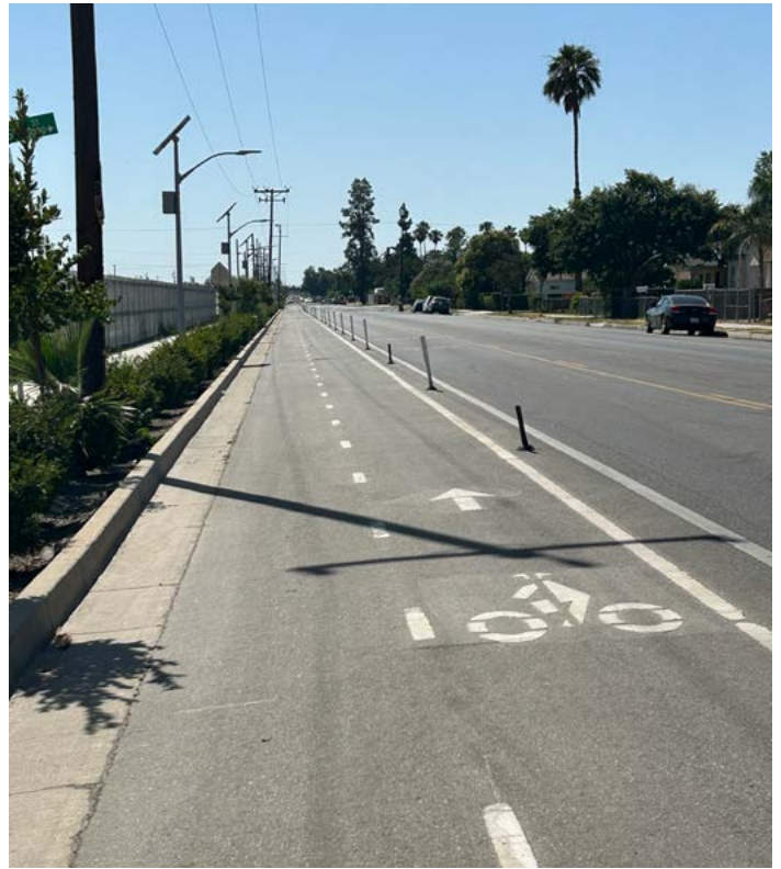
ABOVE: Class IV bike lanes on Kentucky Street provide a safer space in the road separate from motor vehicles.
