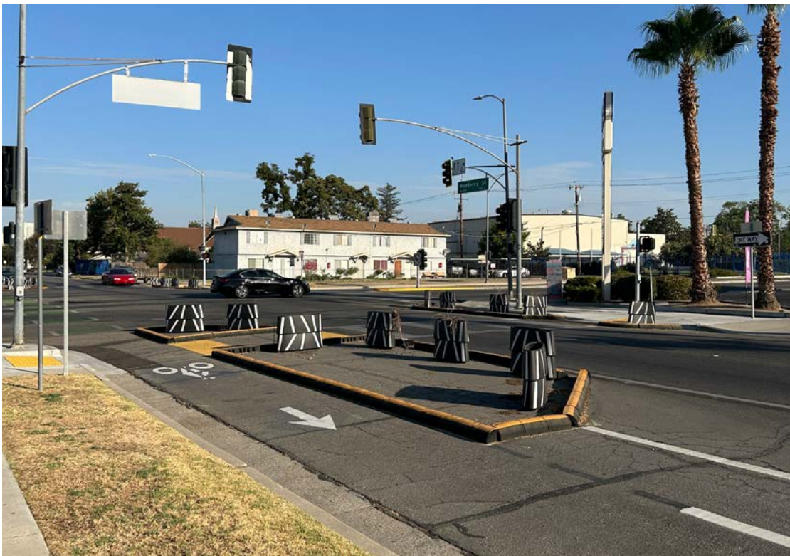
ABOVE: The quick-build curb extensions installed at the Niles Street/Beale Avenue intersection and the Monterey Street/Beale Avenue intersection provide traffic calming measures that slow drivers and enhance crosswalk protection.
