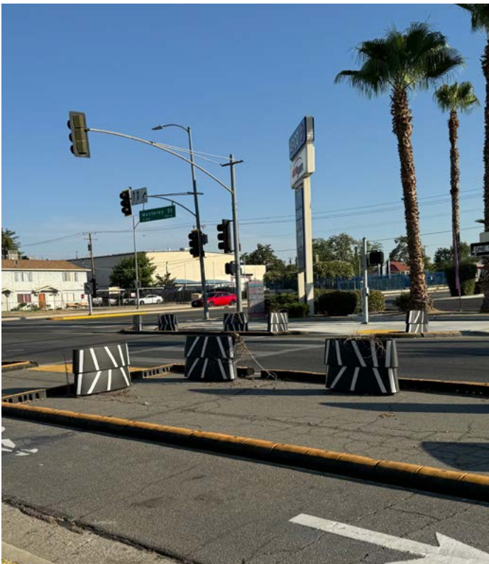
ABOVE: While the quick-build bollards at the Niles Street/Beale Avenue and Monterey Street/Beale Avenue intersections help slow drivers, participants shared that they impact the aesthetic of the intersection.
