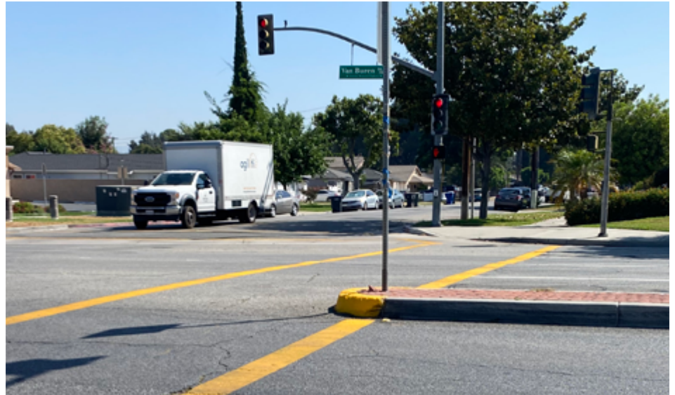
RIGHT: The crosswalk at the Van Buren Boulevard/Garfield Street intersection is partially blocked by the median.
