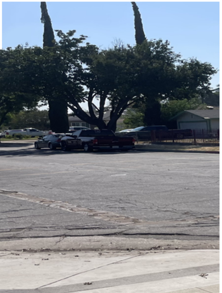
ABOVE: The Home Avenue/Bond Street intersection has faded crosswalks that are low visibility. The road also shows large cracks and is highly uneven, posing a hazard for people walking and biking in the area.
