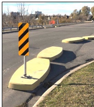
"Temporary Traffic Calming Curbs" (Calgary, AB)
