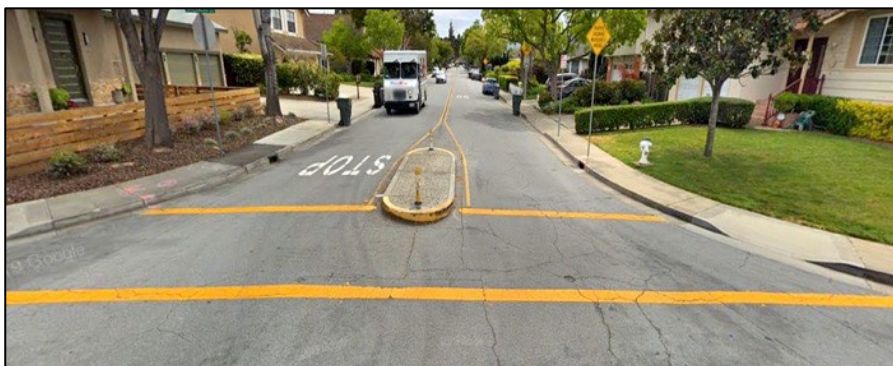
Figure 3-40: Median Island On Residential Street (Canary at Inverness, Sunnyvale CA)
