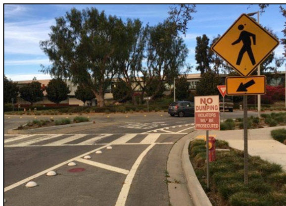
d) NB approach – warning sign upstream of crosswalk. No Dumping sign distracts.
