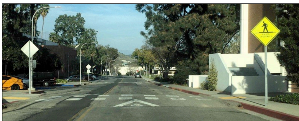
Figure 3-7: Typical Raised Crosswalk With Existing 1-Sided Warning Signs (#5)
