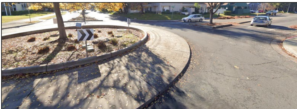
Figure 3-31: Low Raised Truck Apron at Roundabout – Davis CA (Anderson & Alvarado)
