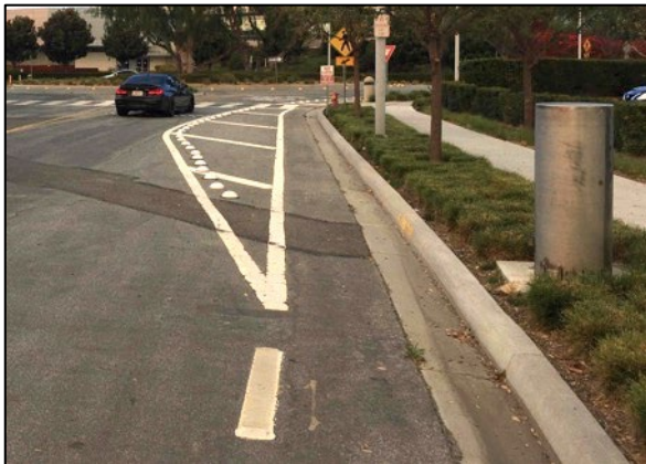
b) NB approach -- merge / bike lane / bypass decision point (no bypass off-ramp)
