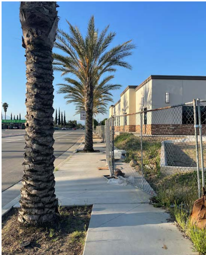
ABOVE: Palm trees along North Walnut Street and current construction significantly reduce the width of sidewalks, make walking along the sidewalks difficult and obstructive to pedestrians and especially to people with limited mobility.
