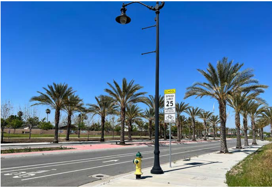
ABOVE: North Walnut Street has a striped and buffered bike lane and pedestrian refuge island.
