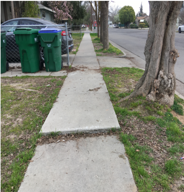
Raised sidewalk on South 4th Street. Sidewalk conditions make it difficult for pedestrians to walk safely especially those traveling with strollers and assistant-mobility devices.
