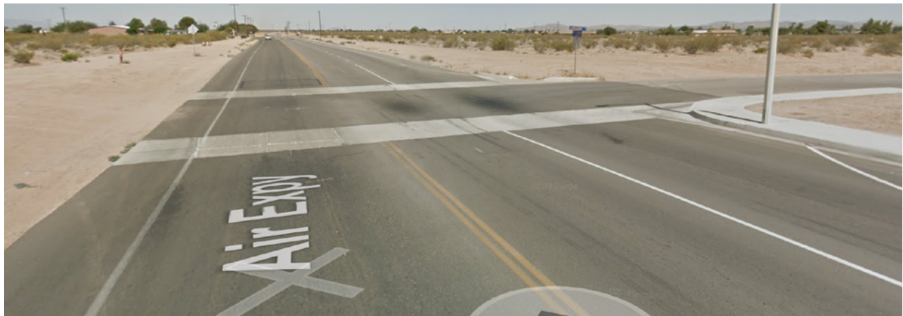
The unmarked crosswalks and unpaved shoulders at the intersection of Air Expressway and Delicious Street create an unsafe crossing for pedestrians and cyclists.
