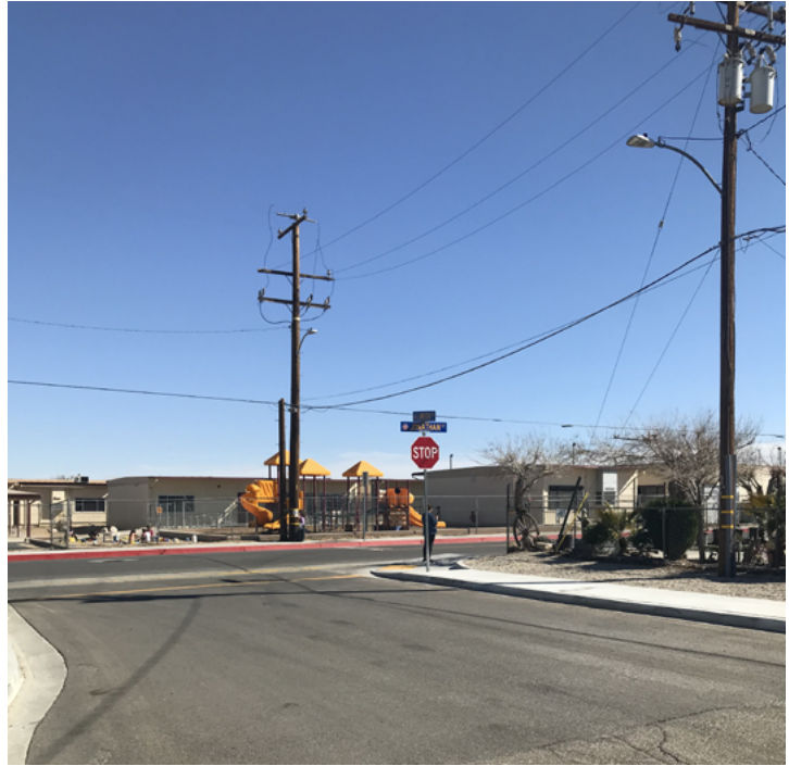
Two street lights in front of Adelanto Elementary School provide all the street lighting at the intersection of Jonathan Street/ Lawson Avenue
