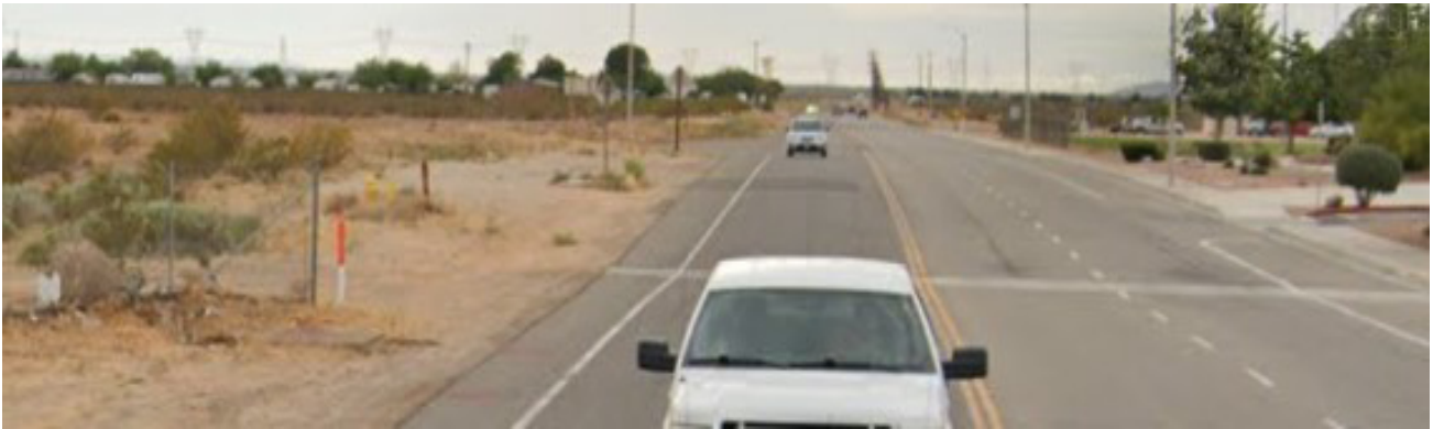
The south side of Air Expressway west of U.S. Route 395 has an unpaved shoulder.
