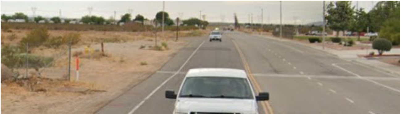
The south side of Air Expressway west of U.S. Route 395 has an unpaved shoulder that is used by pedestrians and bicyclists..
