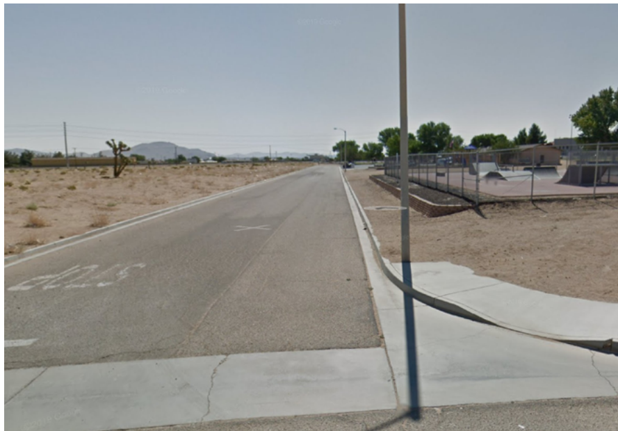
A discontinuous sidewalk along Cortez Avenue leading to the Adelanto Senior Citizens Club.
