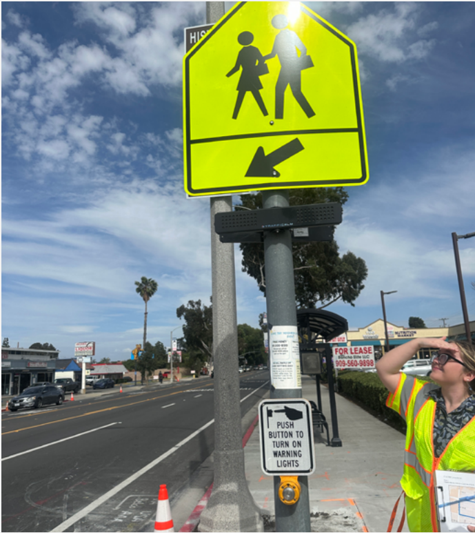
New rectangular rapid flashing beacons (RRFBs) on West Sixth Street help pedestrians cross the street safely.
