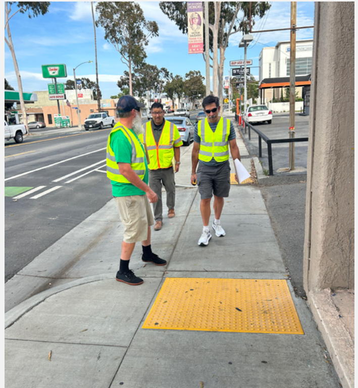
Truncated domes are located on either side of an alleyway exit on West Sixth Street.
