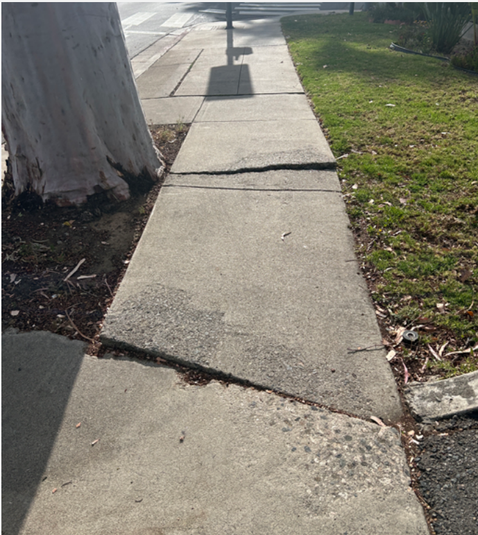
Eucalyptus and palm trees line the West Sixth Street and South Main Street corridors and the roots uplift sidewalks and cause tripping hazards for pedestrians.
