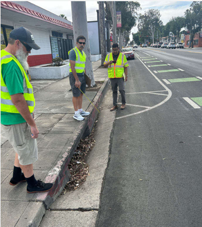
Bicycle paths on the West Sixth Street corridor are obstructed by debris and raised gutter lip posing a hazard for bicyclists.
