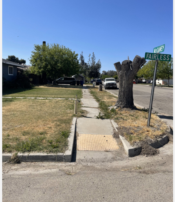
At the West McKamey Avenue/Fairless Avenue intersection, overgrown vegetation obstructs an uneven and cracked sidewalk that abruptly ends at a point further up on West McKamey Avenue.
