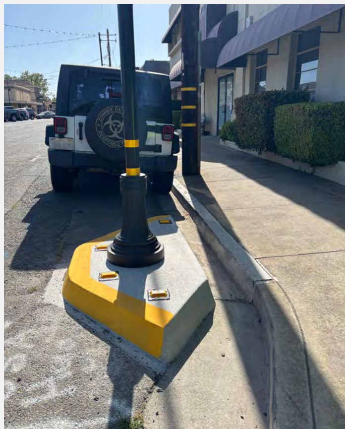
A recently installed structure at the Plumas Street/Teegarden Avenue intersection remains unattached to the curb, leaving a hazardous gap.
