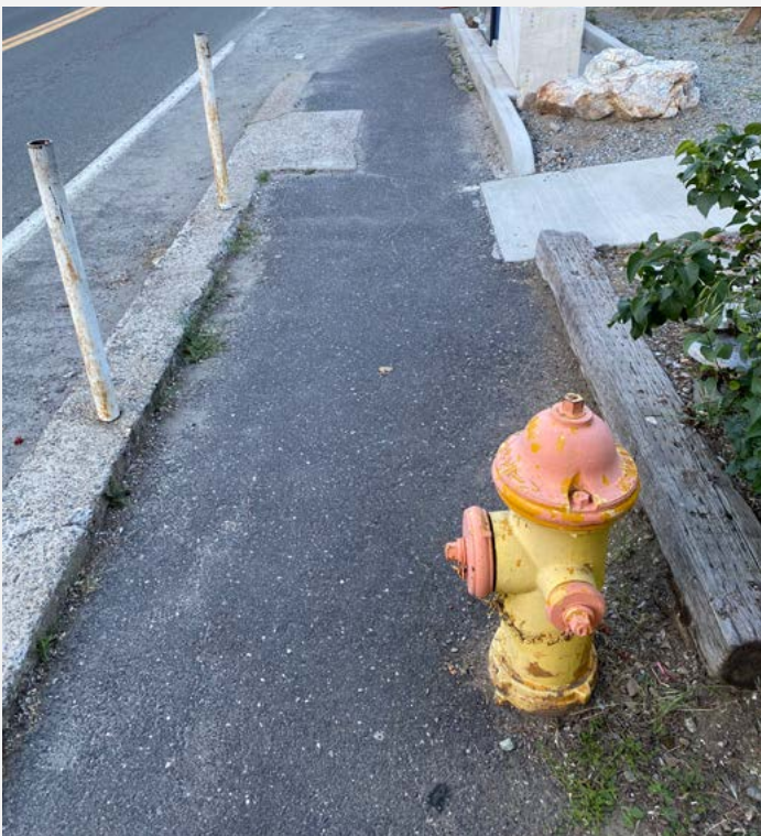
A fire hydrant obstructs the already narrow and short sidewalk in front of Trail Less Traveled.
