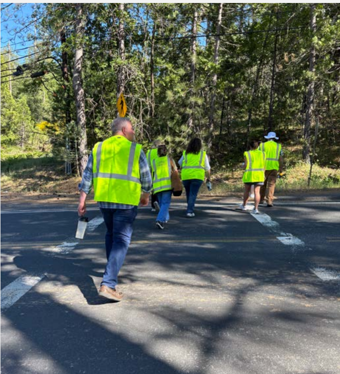
The crosswalk marking outside of GCSD is faded and cracked, making pedestrians less visible to oncoming cars.
