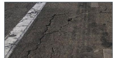
*Unsafe roadway conditions, such as cracked, crumbling uneven pavement along Hardwood Avenue, Avenue J 4, Heaton Avenue, Avenue J 8, and Avenue J contribute to tire damage, falls, and near misses.*
