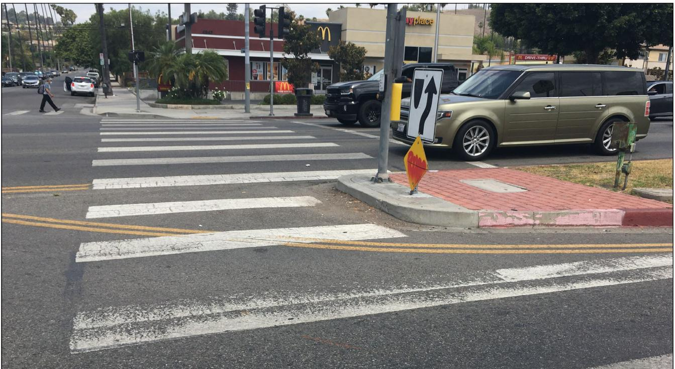
*Huntington Drive is a 6 lane road with a bike lane in both directions. Pedestrians shared that the crossing at the Huntington Drive/Eastern Avenue intersection is difficult due to limited crossing time and a median that is not equipped to be a safe stopping point.*
