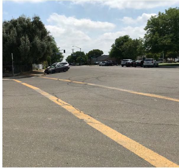
Top Left: Faded conventional crosswalk markings at Castor Avenue/South Orange Avenue.
