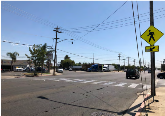
Top Left: Faded conventional crosswalk markings at Castor Avenue/South Orange Avenue.
