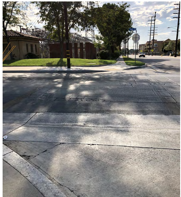
Faded crosswalk markings on West Jackman Street and Fern Avenue.
