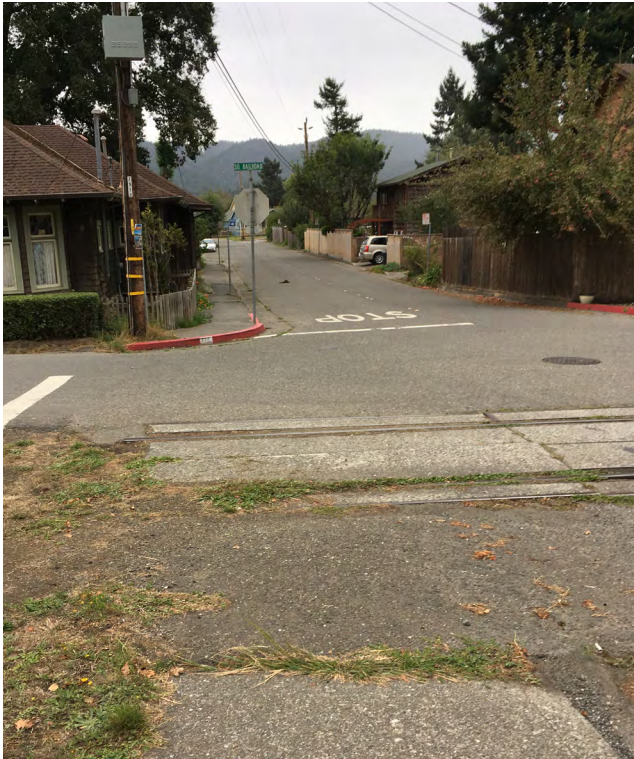
Left: Missing curb ramps at the intersection of Broderick Lane and South Railroad Boulevard.
