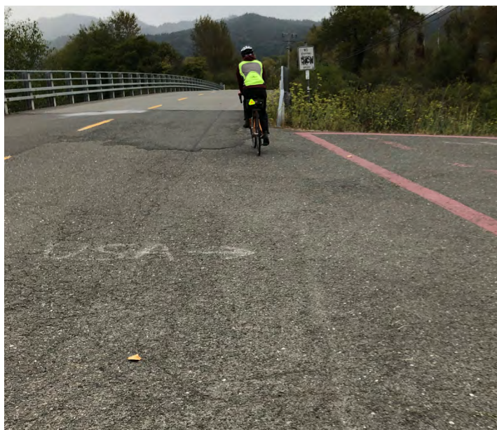
Cracked roadway on Hatchery Road.
