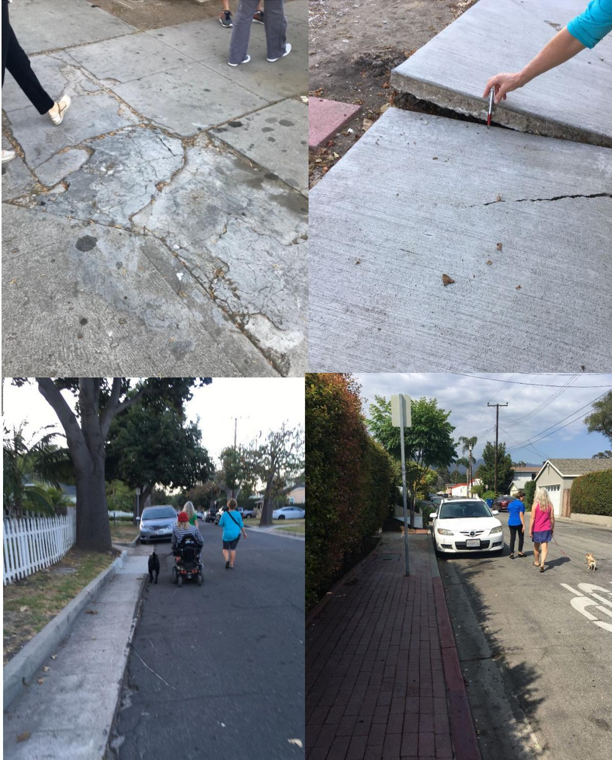
Missing, narrow, upheaved, and cracked sidewalks in the Westside.
