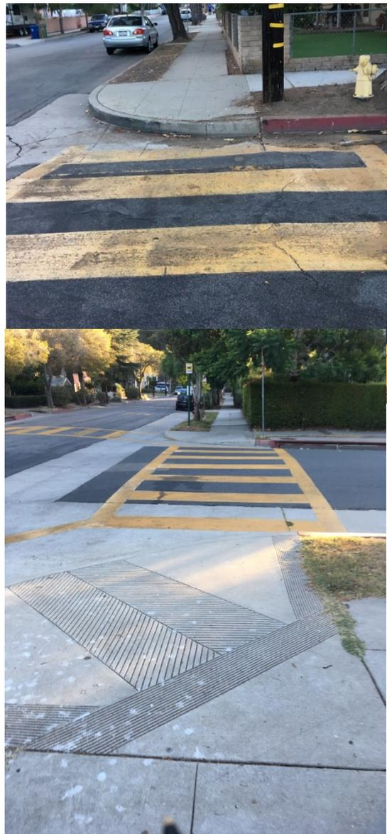
Missing and inconsistent ADA ramps create access and safety challenges for those using assisted mobility devices.
