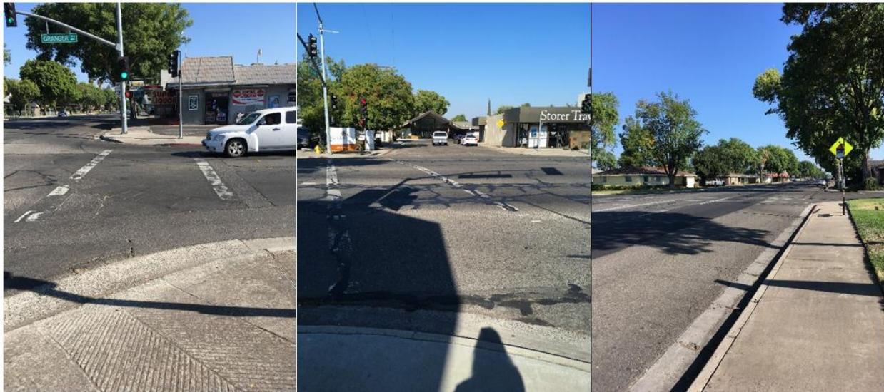
*Faded marked crosswalks along Tully Road traveling towards Granger Avenue and older style apex curb ramps.*
