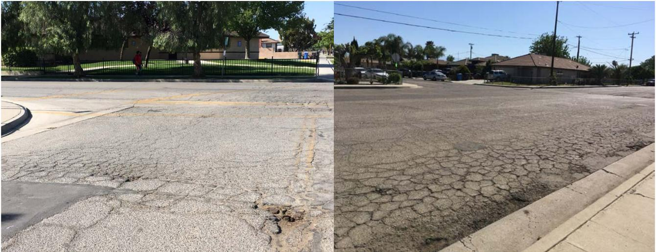
Faded crosswalk and mid-lane markings at the Haven Drive and South A Street intersection near Haven Drive Middle School (left). Cracked and broken pavement along South A Street (right).
