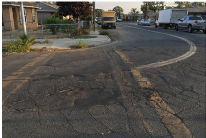
Deteriorating pavement quality and faded markings at S. Santa Clara Avenue & E. Chester Avenue
