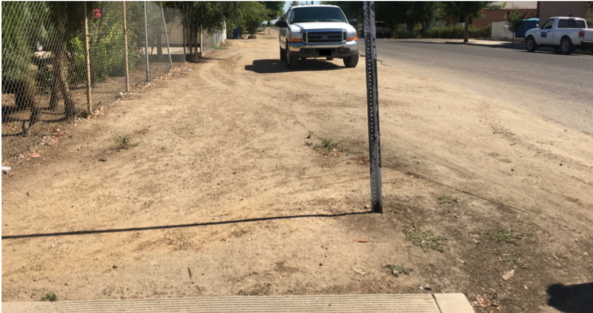
Sidewalks abruptly end in many locations throughout the community.
