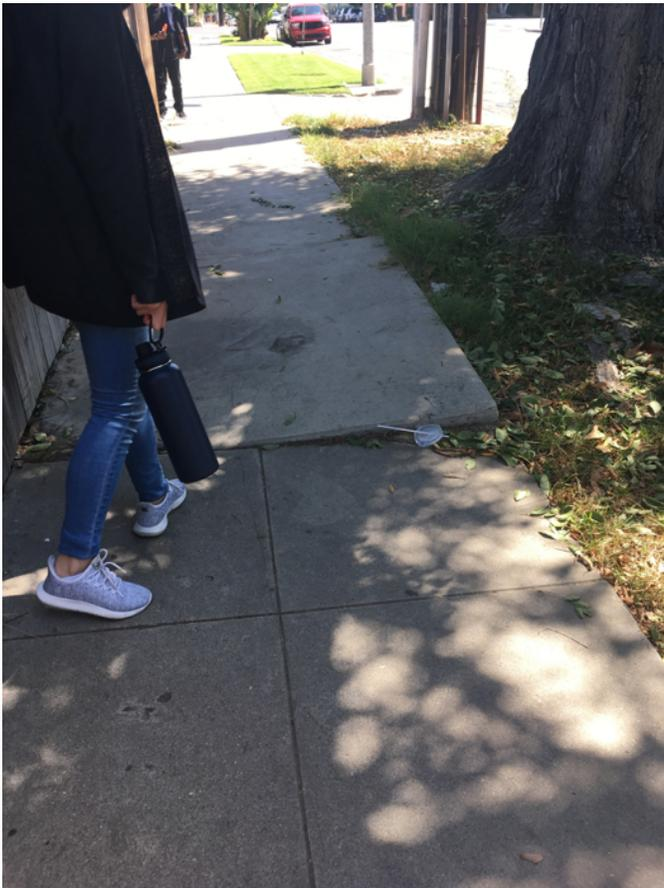
An uplifted sidewalk due to expanding tree roots.
