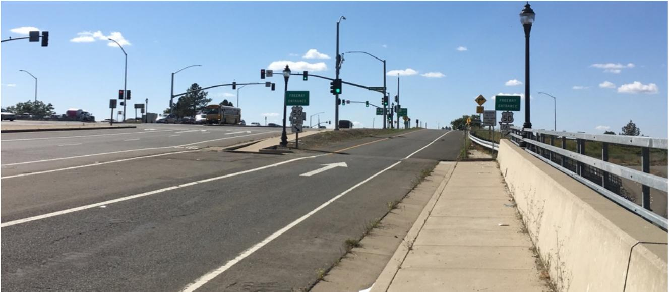
Lack of crosswalk markings or pedestrian warning signage at US 50 on- and off-ramps.
