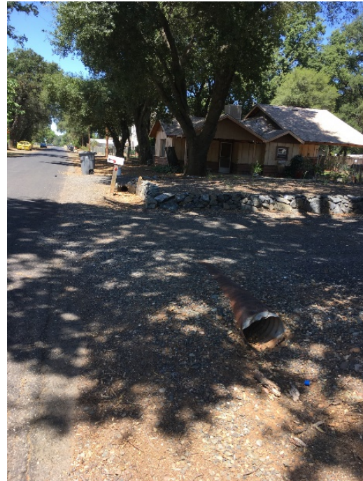
Open drainage canal in an unpaved shoulder in Palermo.
