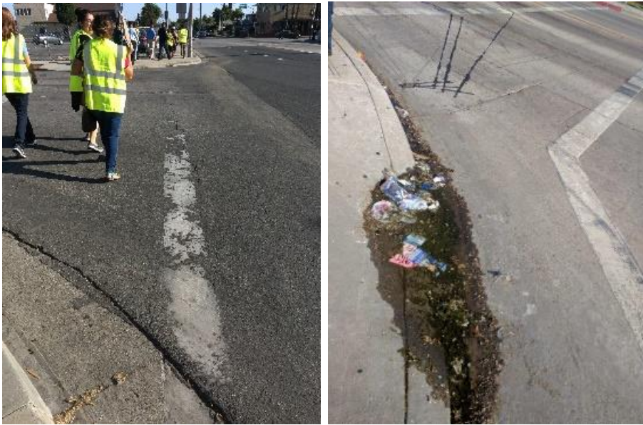
Faded road markings and debris in Florence-Firestone.
